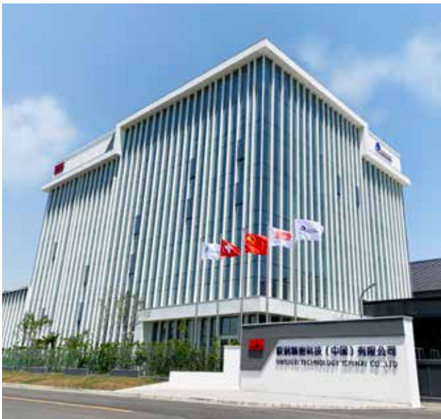
The commissioning of the new production platform in Nantong (China) was completed as planned and will significantly strengthen the competitive position of Electronics.
